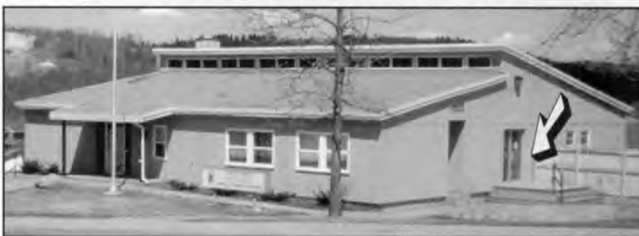
This Saint John police station was bombed on April 23. The bomb was placed on the deck of the side entrance (arrow). Const. Gordon Redburn discovered the bomb and alerted officers inside.
